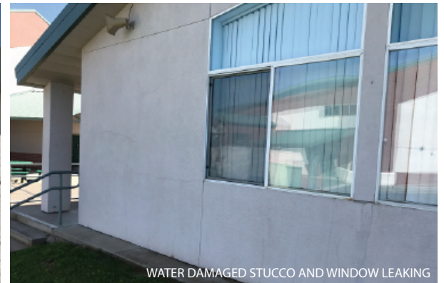
WATER DAMAGED STUCCO AND WINDOW LEAKING
