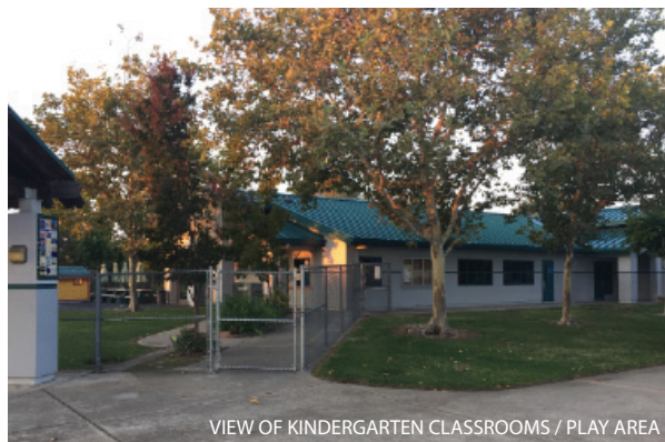
VIEW OF KINDERGARTEN CLASSROOMS / PLAY AREA
