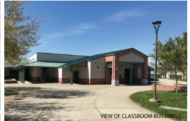
VIEW OF CLASSROOM BUILDING C
