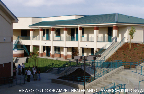
VIEW OF OUTDOOR AMPHITHEATER AND CLASSROOM BUILDING A
