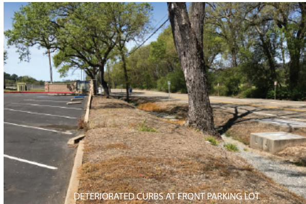
DETERIORATED CURBS AT FRONT PARKING LOT
