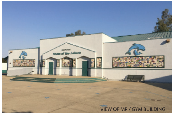
VIEW OF MP / GYM BUILDING
