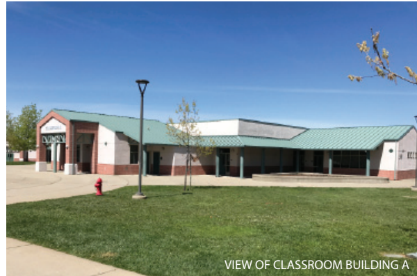
VIEW OF CLASSROOM BUILDING A
