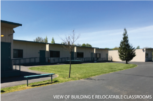
VIEW OF BUILDING E RELOCATABLE CLASSROOMS
