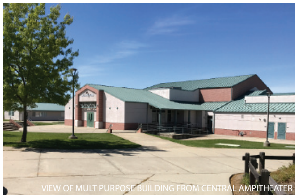
VIEW OF MULTIPURPOSE BUILDING FROM CENTRAL AMPITHEATER
