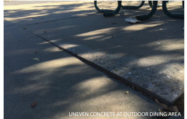
UNEVEN CONCRETE AT OUTDOOR DINING AREA
