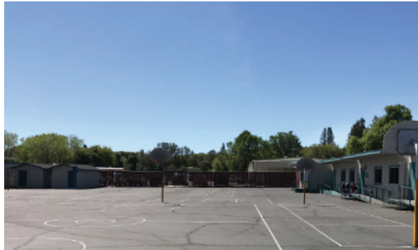
NEW KINDERGARTEN BUILDING DOES NOT MATCH LOOK OF EXISTING
