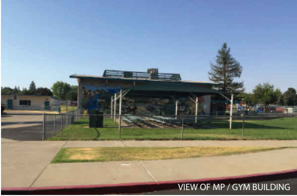
VIEW OF MP / GYM BUILDING
