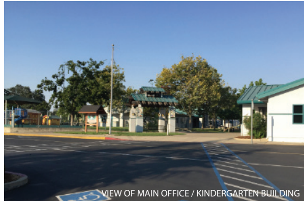
VIEW OF MAIN OFFICE / KINDERGARTEN BUILDING
