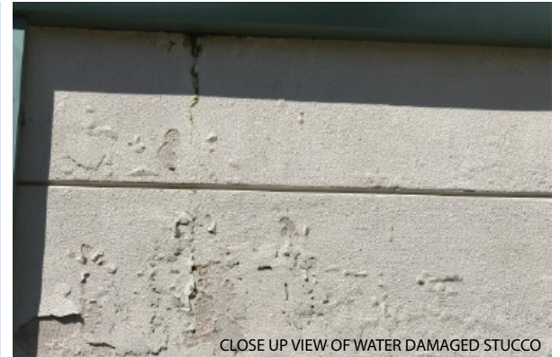
CLOSE UP VIEW OF WATER DAMAGED STUCCO
