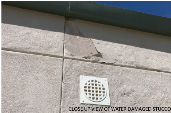
CLOSE UP VIEW OF WATER DAMAGED STUCCO
