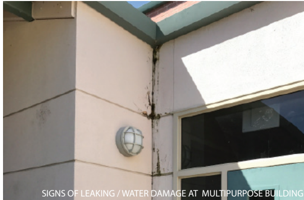
SIGNS OF LEAKING / WATER DAMAGE AT MULTIPURPOSE BUILDING
