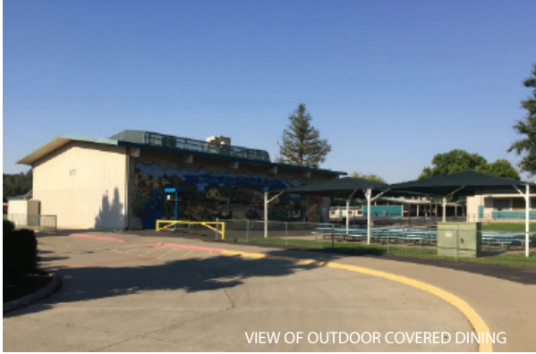
VIEW OF OUTDOOR COVERED DINING
