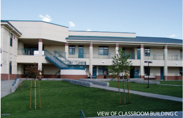
VIEW OF CLASSROOM BUILDING C
