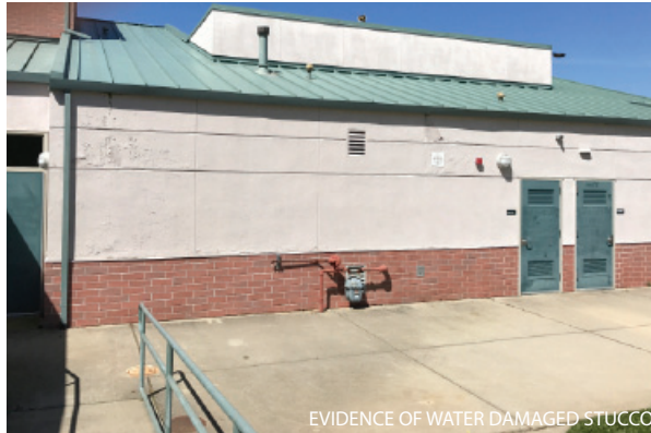
EVIDENCE OF WATER DAMAGED STUCCO
